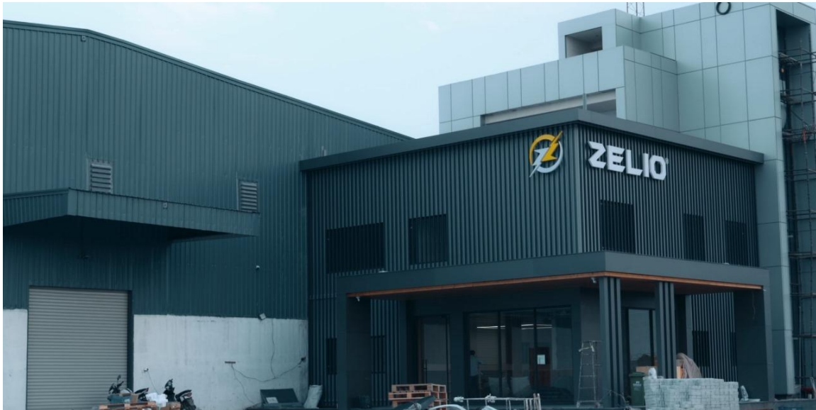
(Current Manufacturing unit located at Ladwa, Hisar (outside view))
